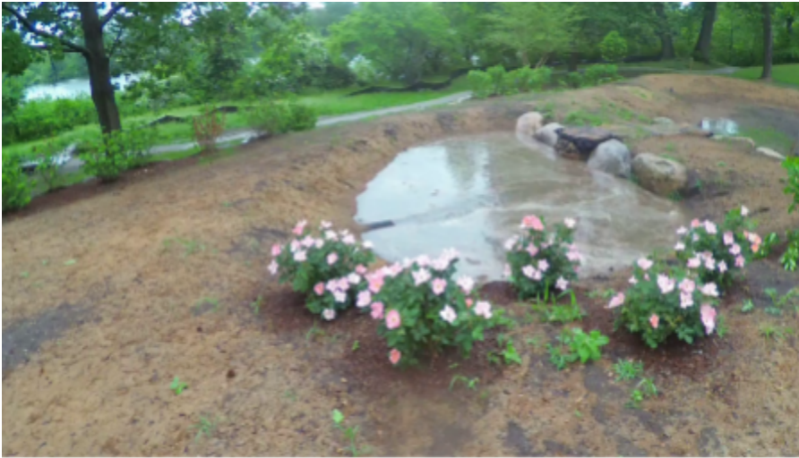
An infiltration basin in Roger Williams Park, functioning as designed, during a rain event in 2021.
