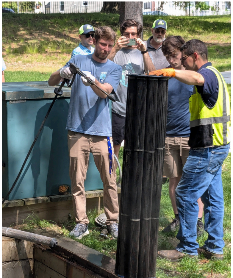
Bottom Right: Christopher Dill with RIDEM and Nate Marles power washing a filter cartridge
