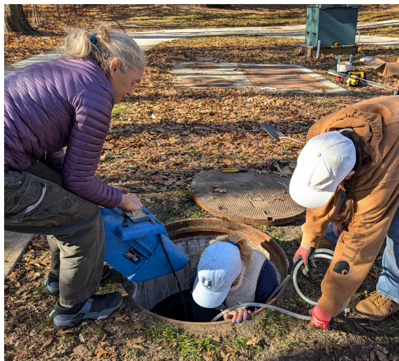
Madison, Q and Sophia installing monitoring equipment at the treatment train
