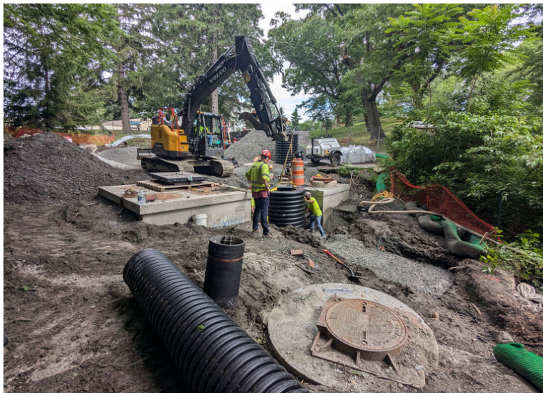
Treatment Train construction photo
