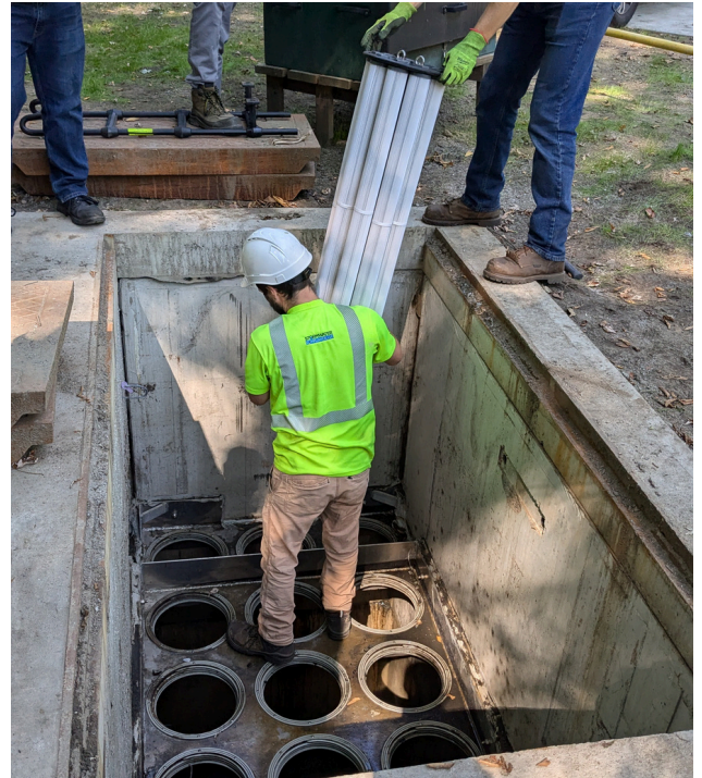
Stormwater Compliance installing jellyfish filter cartridges.
