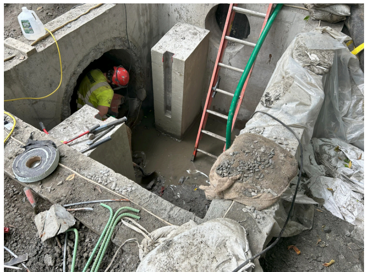
Inside the treatment train diversion structure during construction
